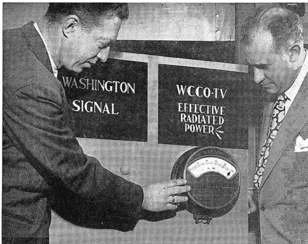
FIG. 3. Shown (l. to r.) are Neil B. Coil, Transmitter Supervisor and John M. Sherman, the author, checking the output meter which indicates 100 kw power.
