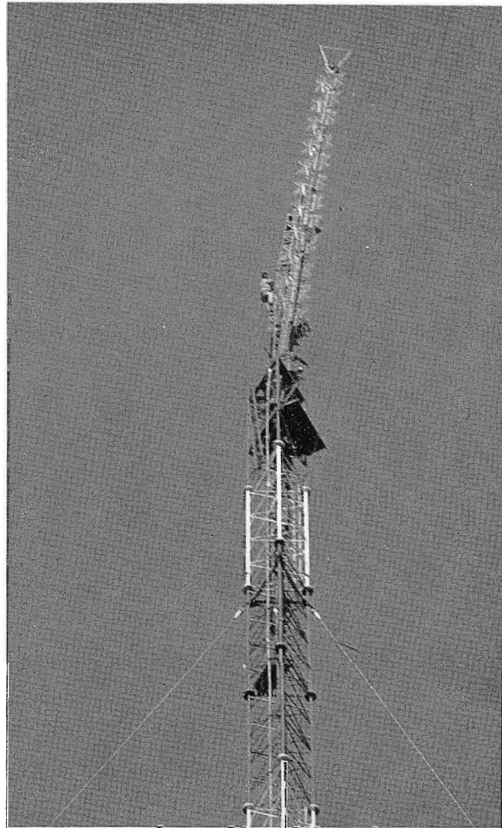
FIG. 4. Resting atop the 500-foot tower, the antenna is being prepared for its final vertical mounting. The specially-constructed steel gin pole can be seen at the lower left side of the antenna before its separation.
