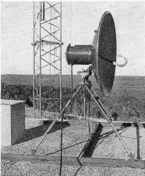
FIG. 10. Microwave studio-transmitter link. Photo shows parabolic receiving antenna on transmitter building roof. Transmitting antenna is mounted on Driskill Hotel roof—studio location in downtown Austin.
